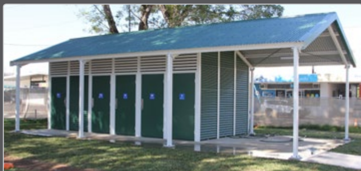
Image above: Olympus Custom Shelter Toilet Buildings for Hinchinbrook Council. This project included a service area which is located at the back of the building and incorporates hidden cisterns.
